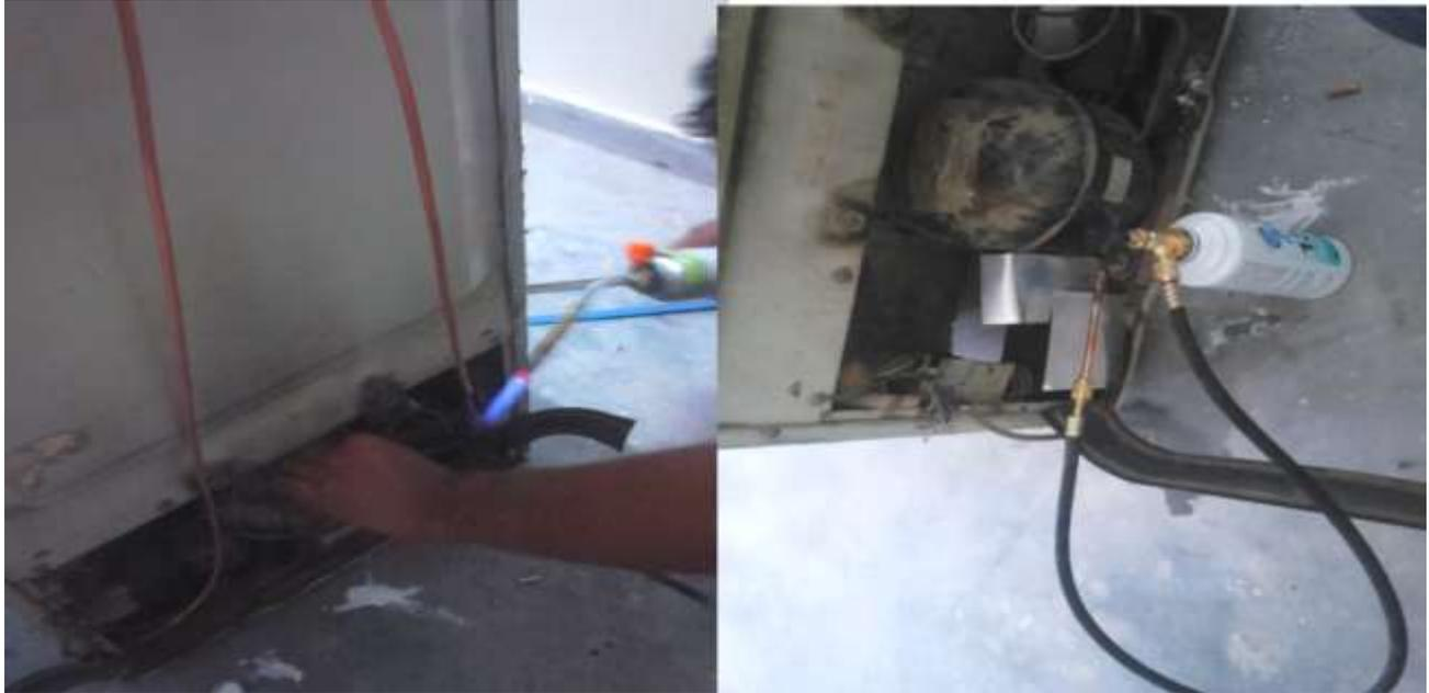
**Fig 1.4: Welding of copper tubes and gas filling by cylinder.**
