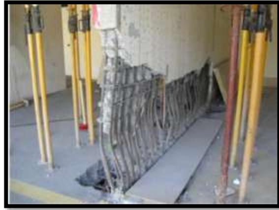
Figure 2. First storey buckling in Chile earthquake [2]
