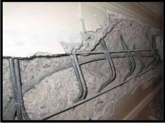
Figure 1. Buckling of longitudinal reinforcement
